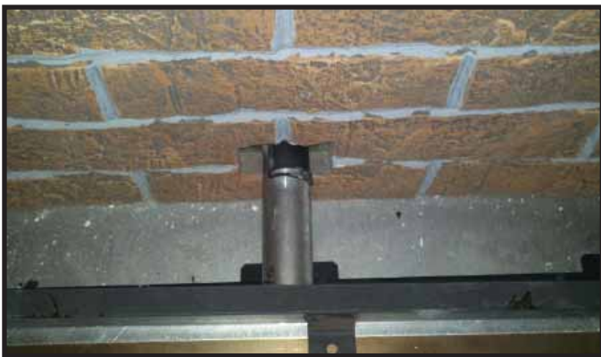
Figure 14.14 Air Shutter
